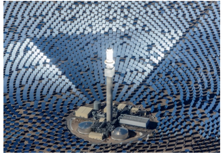
Gemasolar solar power plant (Spain)
