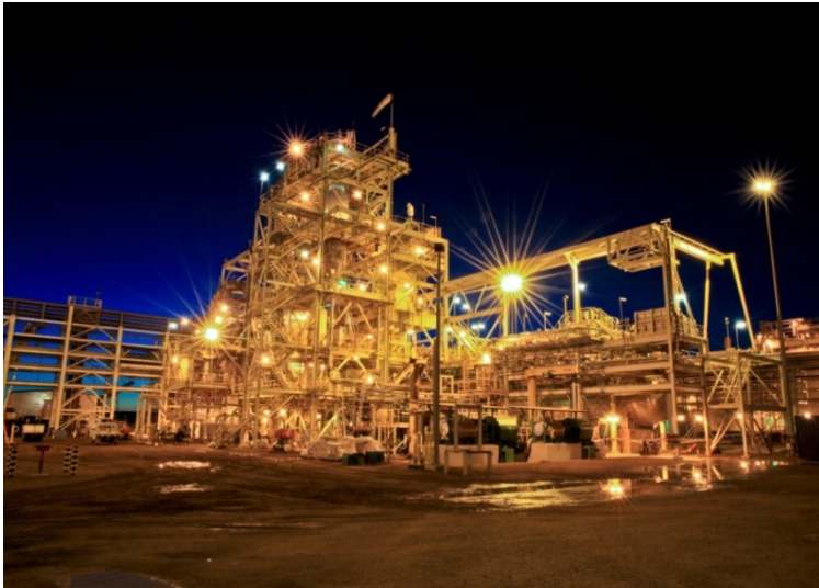
Ravensthorpe Nickel Operation plant (WA)
